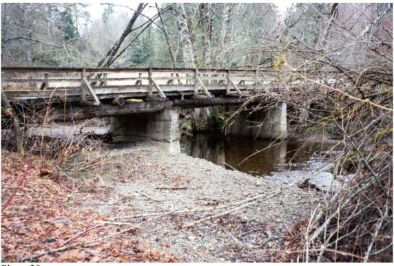
Photo 30. River confinement and gravel deposition subsequent to bridge crossing on North fork.
