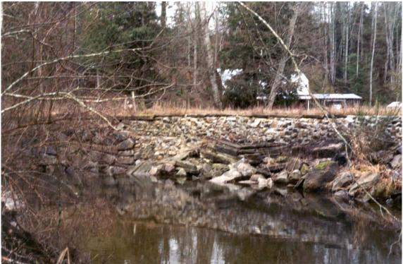
Photo 9. Cement wall constructed to armour bank.
