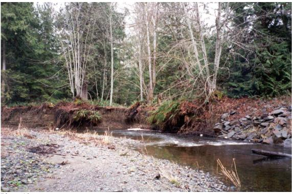
Photo 10. Armouring the bank can move or increase erosion downstream.
