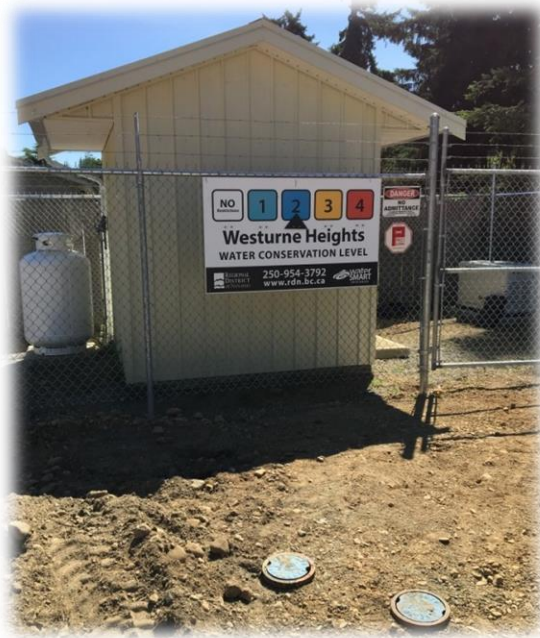
Westurne Heights Pumphouse and Buried Cisterns
