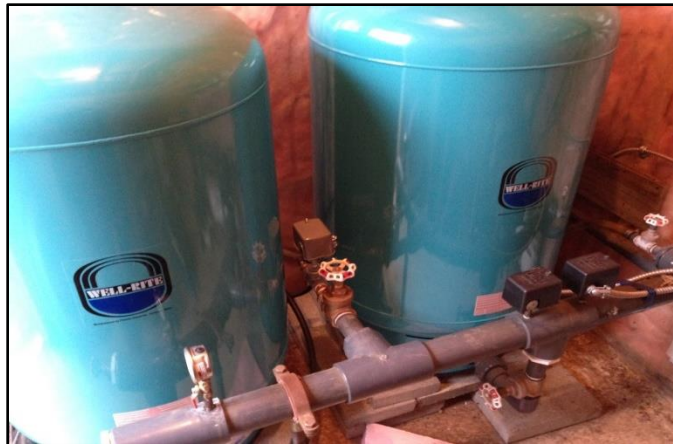
Pressure tanks in the pump house
