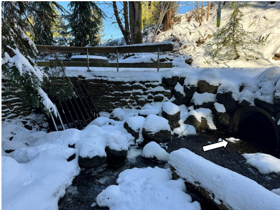
Figure 2. Inlet of culverts (including daylighting system) under Crescent Road at Grandon Creek Trail Park (culvert with grate accommodates high flows). Arrow indicates flow direction. Photograph collected February 12, 2025.
