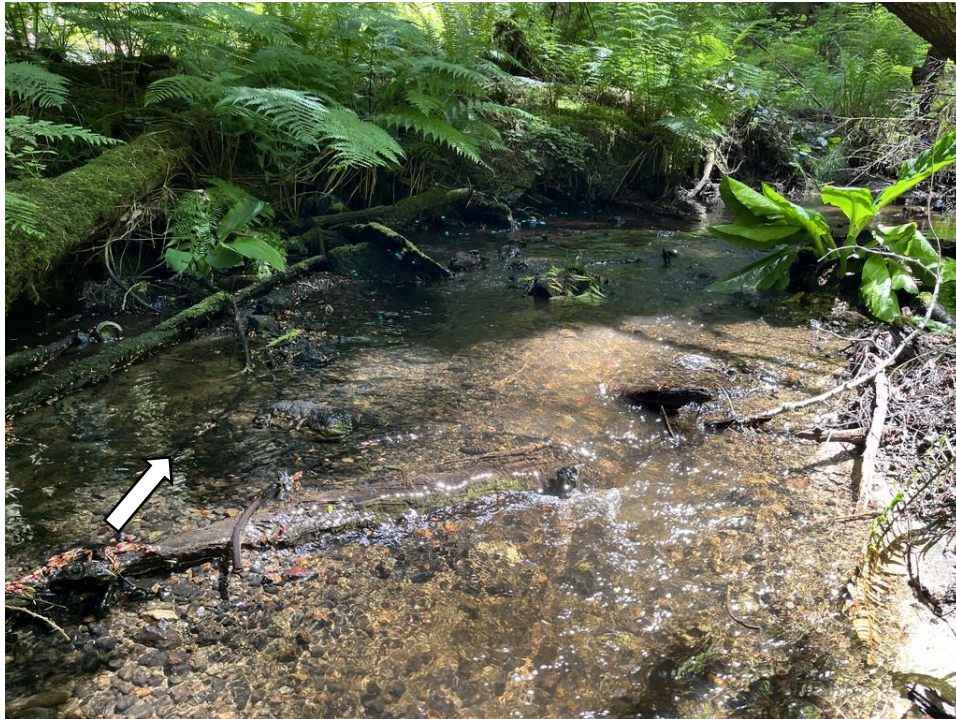
Figure 12. Perched culvert from Village Way roadside ditching. Culvert drop is 2.6 m (fish barrier). Arrow indicates flow direction. Photograph collected June 7, 2024.
