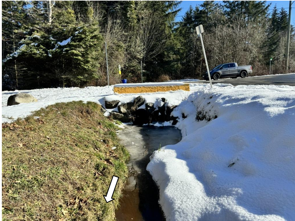
Figure 12. River right tributary culvert outflow under rail line. Arrow indicates flow direction. Photograph collected February 12, 2025
