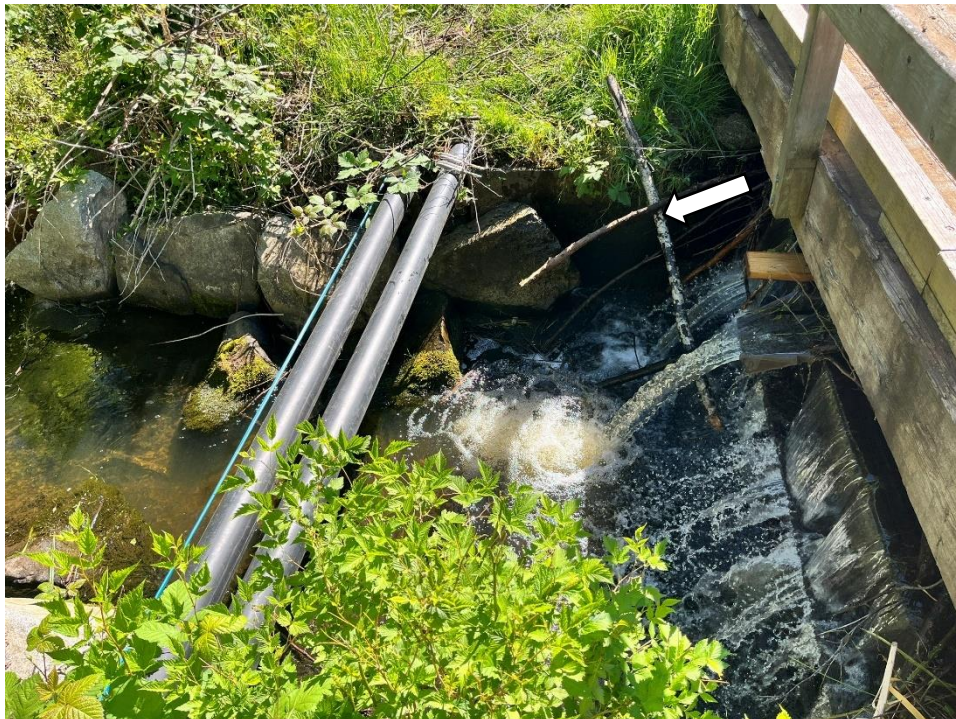
Figure 4. Outlet from Golf Course pond beneath foot bridge: drop of ~1 m, though the drop is reduced to 0.8 m with boards removed (fish-passable). Arrow indicates flow direction. Photograph collected June 7, 2024.
