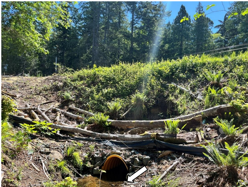
Figure 8. Outlet of culvert under Crescent Road E. Riparian remediation planting and sediment and erosion control measures in place. Arrow indicates flow direction. Photograph collected June 7, 2024.
