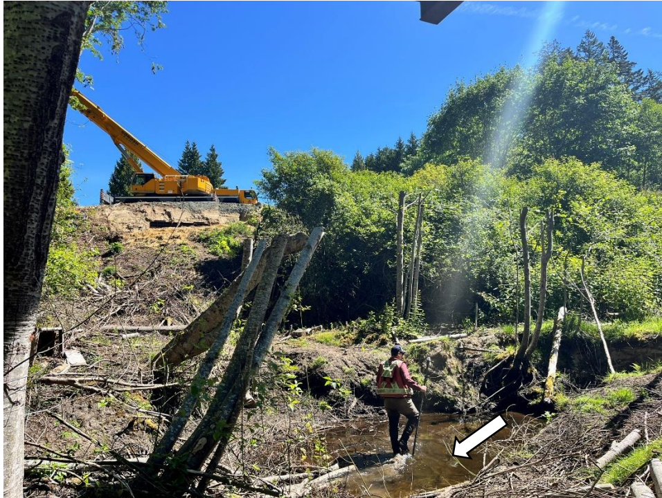
Figure 8. Outlet of culvert under Crescent Road E. Riparian remediation planting and sediment and erosion control measures in place. Arrow indicates flow direction. Photograph collected June 7, 2024.
