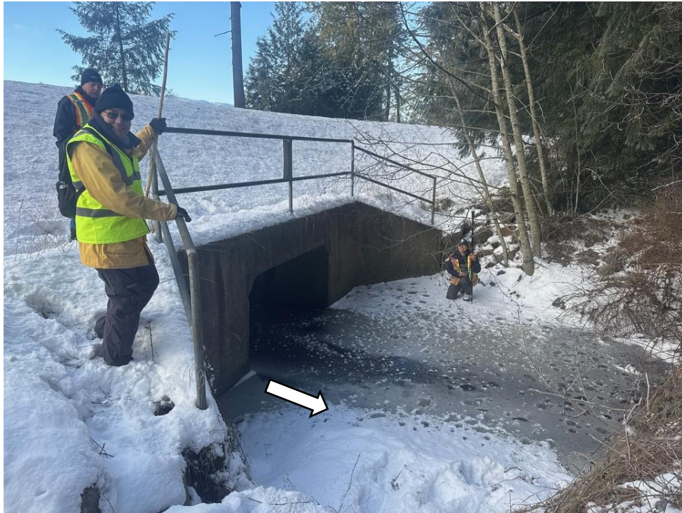
Figure 22. Rupert Road box culvert inflow. Arrow indicates flow direction. Photograph collected February 26, 2025.
