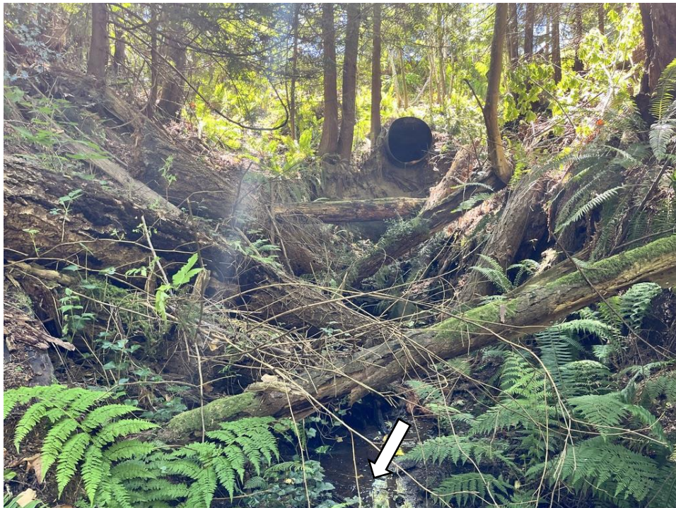
Figure 12. Perched culvert from Village Way roadside ditching. Culvert drop is 2.6 m (fish barrier). Arrow indicates flow direction. Photograph collected June 7, 2024.
