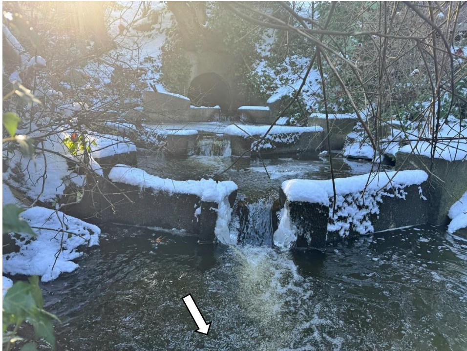
Figure 2. Inlet of culverts (including daylighting system) under Crescent Road at Grandon Creek Trail Park (culvert with grate accommodates high flows). Arrow indicates flow direction. Photograph collected February 12, 2025.
