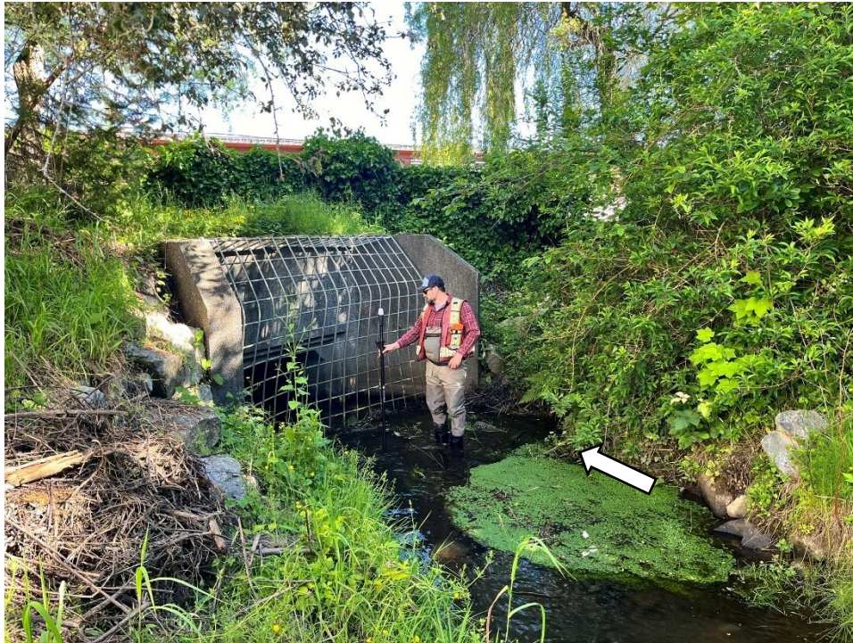
Figure 4. Outlet from Golf Course pond beneath foot bridge: drop of ~1 m, though the drop is reduced to 0.8 m with boards removed (fish-passable). Arrow indicates flow direction. Photograph collected June 7, 2024.
