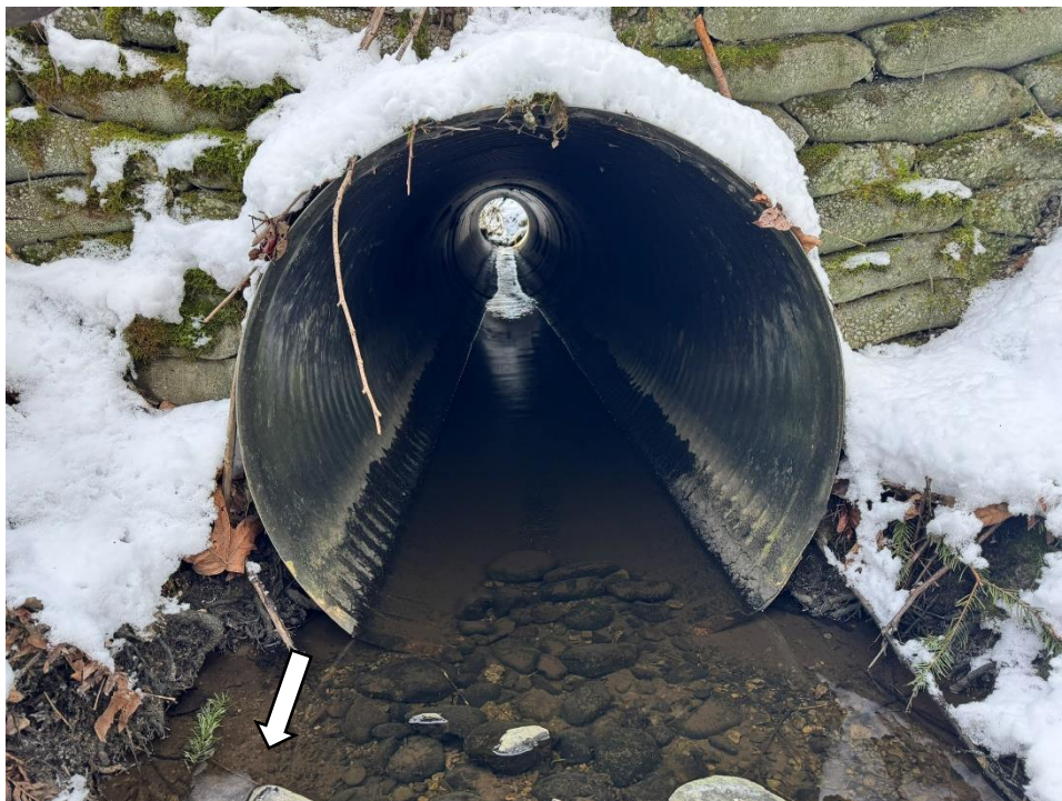
Figure 12. River right tributary culvert outflow under rail line. Arrow indicates flow direction. Photograph collected February 12, 2025
