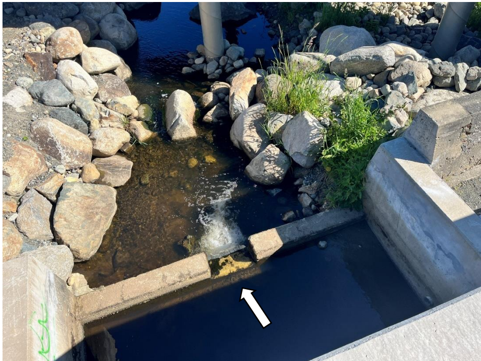
Figure 2. Outlet of Beach Creek under Hwy 19A, including fish-passable weirs. Arrow indicates flow direction. Photograph collected June 7, 2024.
