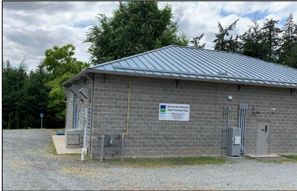
Nanoose Bay Water Treatment Plant
