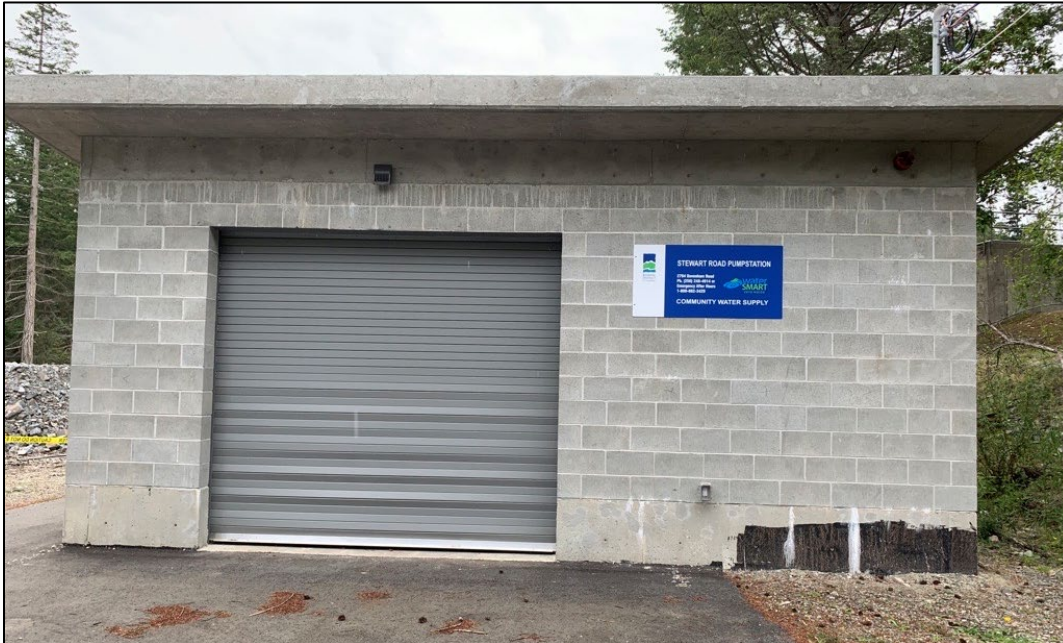
Stewart Road Pump Station (2020)
