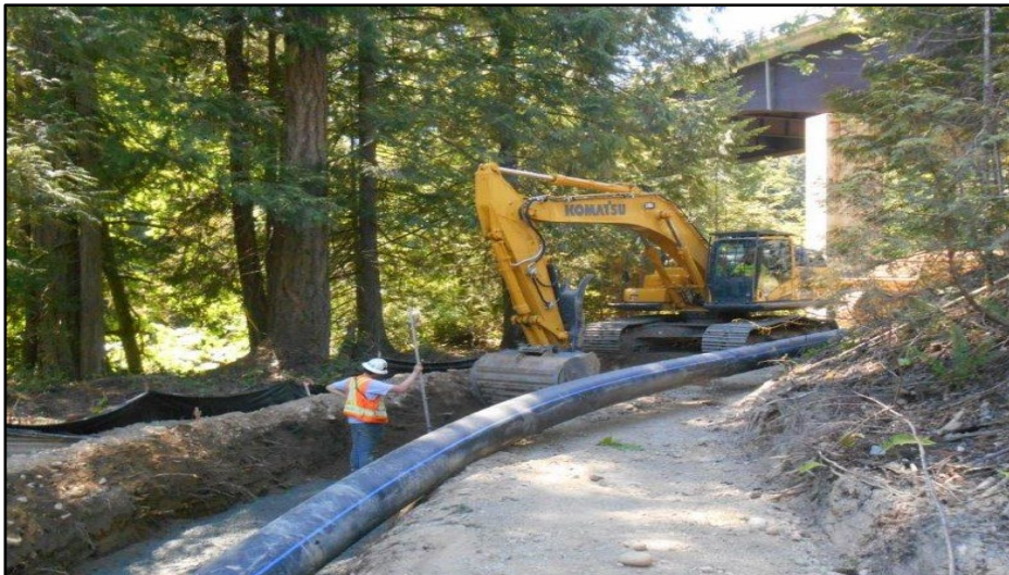
ERWS Bulk Water Transmission Line Construction near Hwy 19 (2017)
