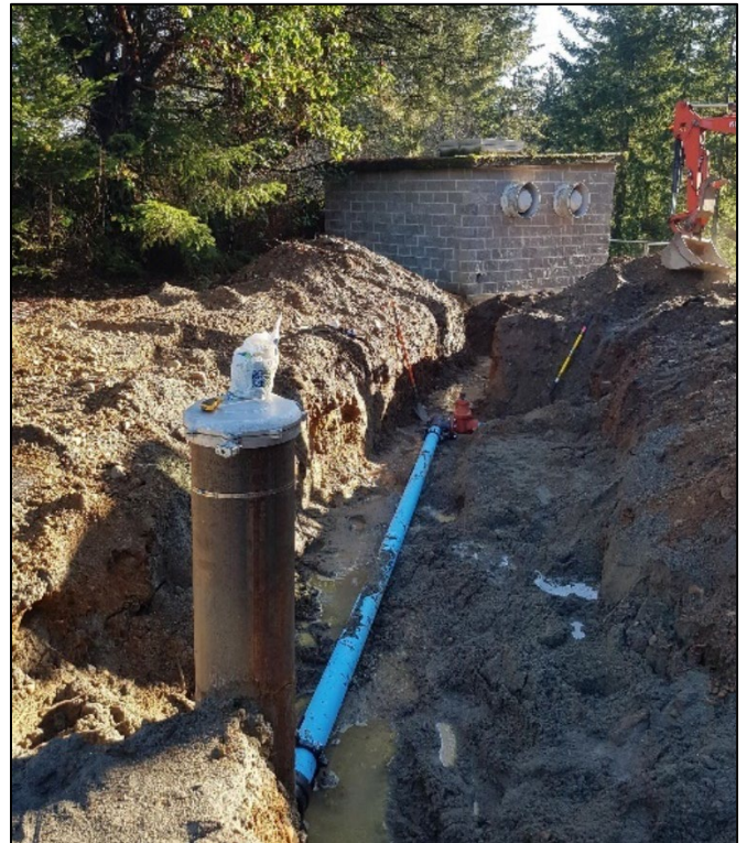
West Bay Well #5 and pitless adaptor being installed (2024)
