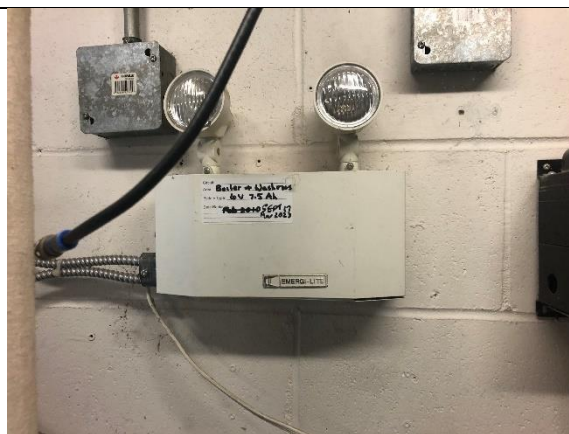
Sample: Visual identification Location: Room 26 Description: Emergency light Hazardous Material: Batteries
