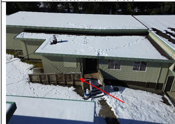
Sample: Visual identification Location: Exterior front entrance Description: Pressure treated wood Hazardous Material: Arsenic (potential)
