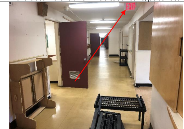
Sample: Visual identification Location: Room 5 Description: Exit sign Hazardous Material: Batteries
