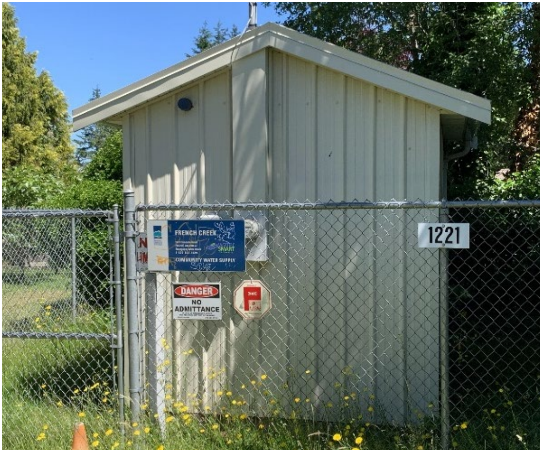
French Creek Well #2 pumphouse
