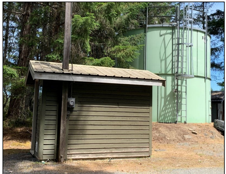
Decourcey Pumphouse and Water Storage Reservoir
