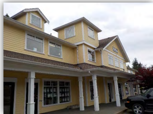
Rooflines & exterior architectural design detail.
