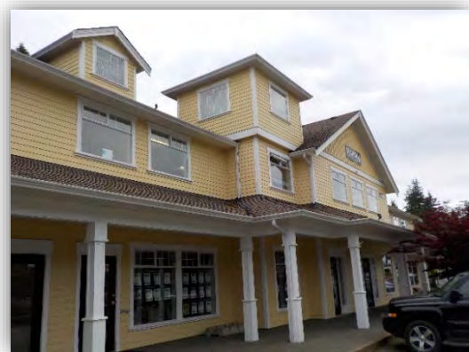
Rooflines & exterior architectural design detail.
