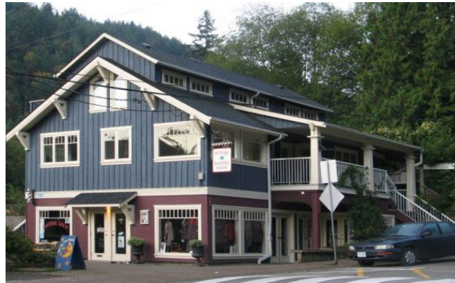
Example of third floor space built into the roofscape.
