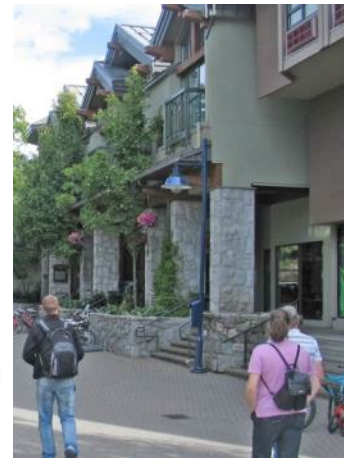
Example of a covered walkway
