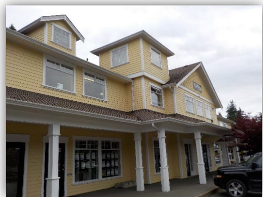
Rooflines & exterior architectural design detail.
