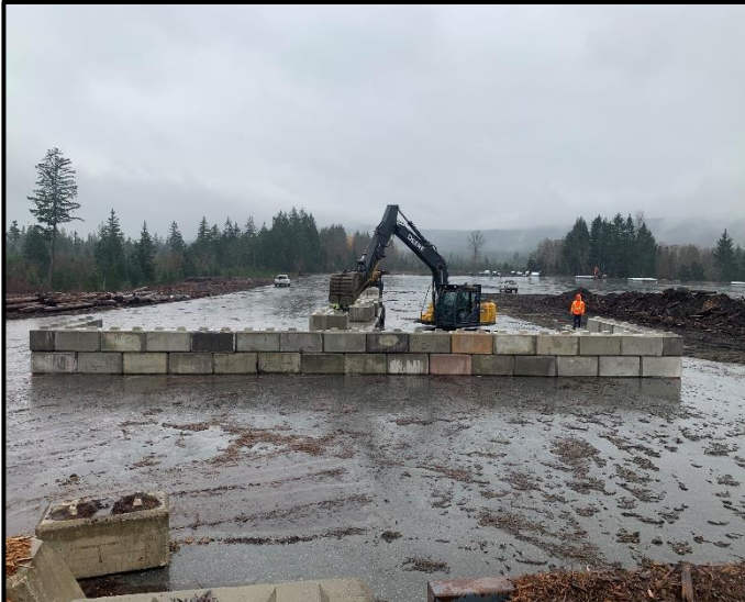
Photograph 3: Stockpile at Blackjack constructed using concrete lock blocks. (November 2021)
