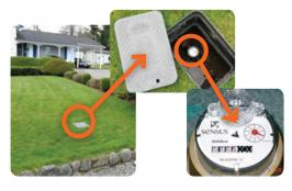
Reading your water meter: Look at the meter face. Is the leak detector (usually a black triangle or red star) moving? If so, and all sources of water in the house have been shut off, you have a leak.
