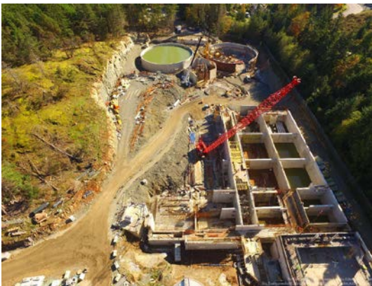
Photo left: Secondary treatment area – bioreactors and clarifiers
