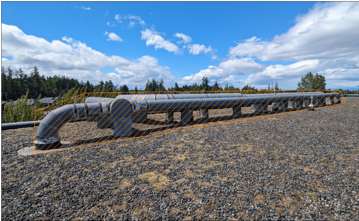
3 DEHUMIDIFIER DUCTWORK KEYNOTES: DEMOLISH DEHUMIDIFIER DUCTWORK ON ROOF AND INSIDE RINKS.
