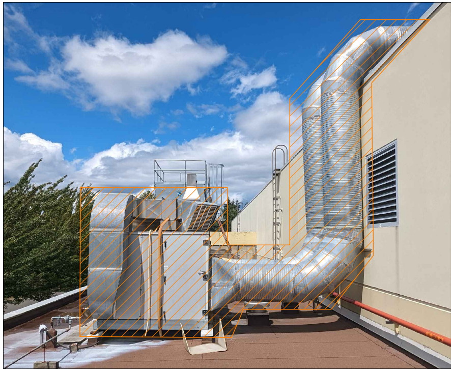
2 EXISTING DEHUMIDIFIER KEYNOTES: DEMOLISH EXISTING DEHUMIDIFIER AND DUCTWORK.
