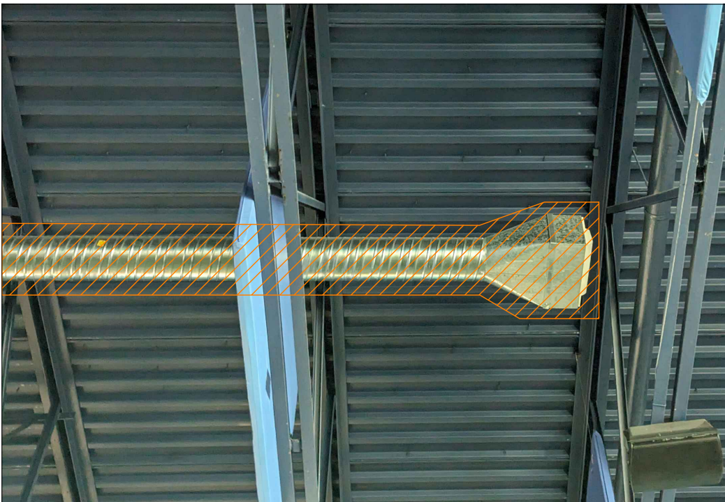
8 DEHUMIDIFIER DUCTWORK IN THE POND KEYNOTES: DEMOLISH DEHUMIDIFIER DUCTWORK IN THE POND AND PATCH PENETRATIONS
