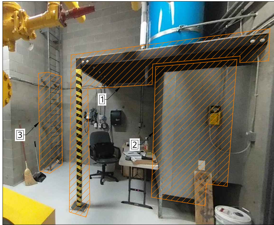
1 MECHANICAL ROOM PLATFORM KEYNOTES: DEMOLISH EXISTING PLATFORM AND REPLACE (SEE STRUCTURAL FOR DETAILS). TRIM BACK DUCTWORK AND MOVE CONTROL DAMPER CLOSER TO WALL. DEMOLISH LOWER HALF OF LADDER TO HEIGHT OF NEW PLATFORM.
