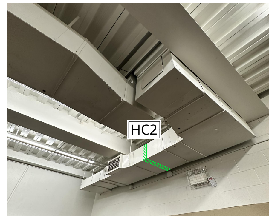
6 HEATING COIL (HC2) LOCATION IN SUPPLY DUCT
