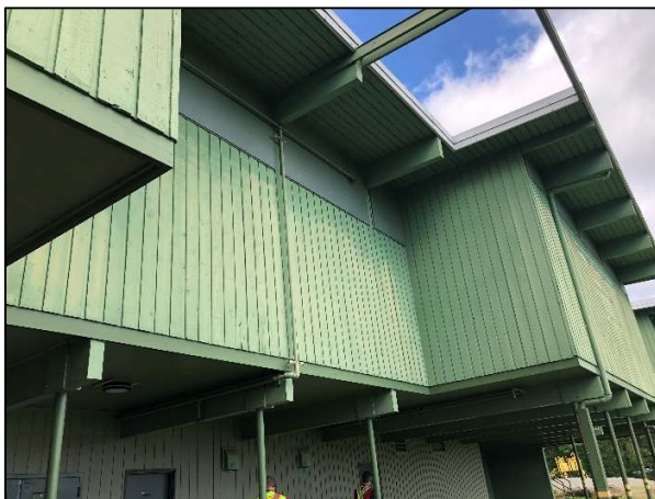
Photo 3 - Exterior wall paint has faded
