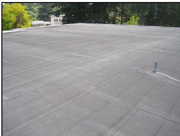
SBS Modified Bitumen Membrane Renewal
