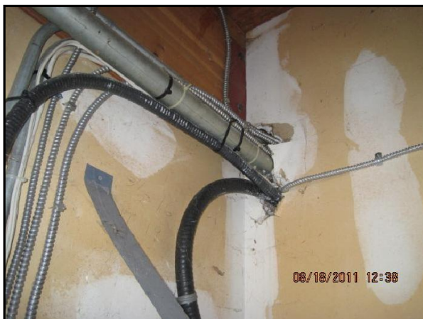
Electrical Conduits - Fire Stopping Not Installed
