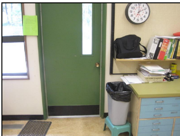
Interior Doors - Hardware Not Accessible
