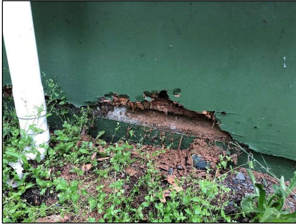
Photo 5 - Deterioration of painted plywood at base of wall due to close proximity to ground surfaces
