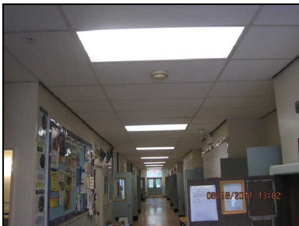
Non-Seismic Luminaire - Corridors
