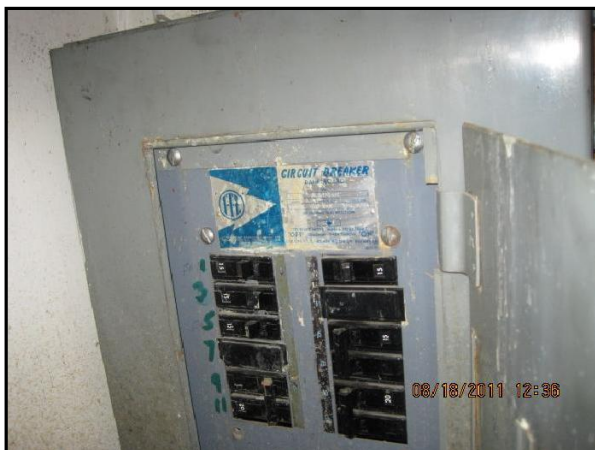
Panelboards, Feeders and Disconnects - 120/240V Renewal
