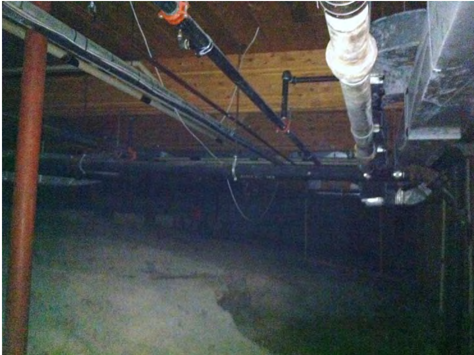
View of crawlspace behind basement storage areas. Note rock slope and lack of interior bearing walls.
