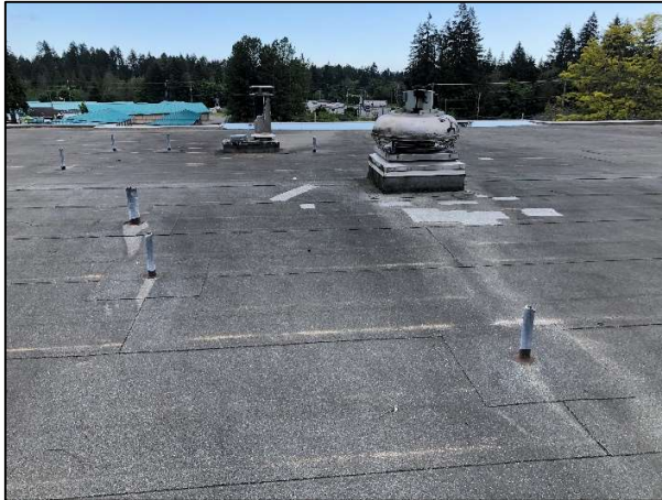
Photo 1 - View of primary roof shows degradation and patch repairs
