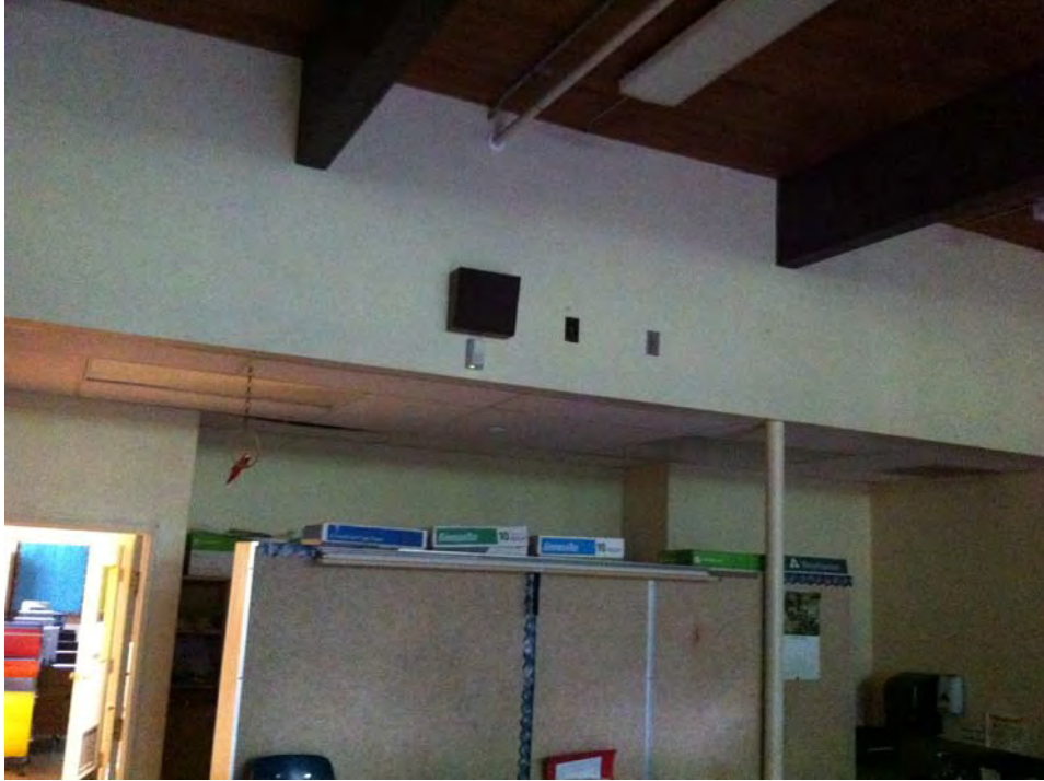
Interior view of classroom looking towards corridor showing supporting pipe column
