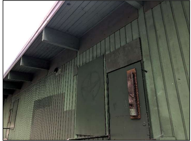
Photo 6 - Overall, the cedar cladding appears to be in good condition.
