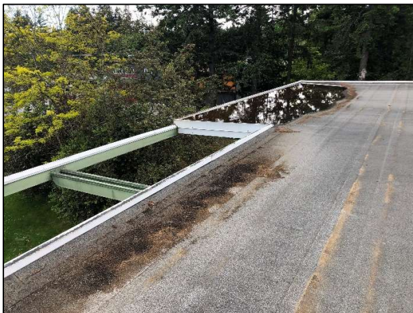
Photo 3 - Ponding and staining
