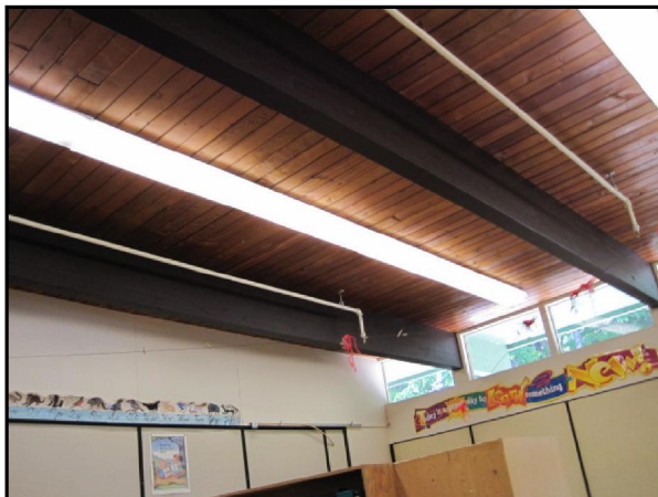
Fire Protection - Sprinkler Piping - No Seismic Restraint
