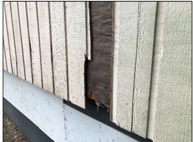
Photo 2 - Vertical painted cedar cladding installed over building paper
