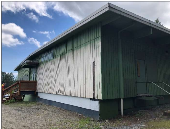
Photo 1 - North-West corner of building shows where the building was painted around a portable.
