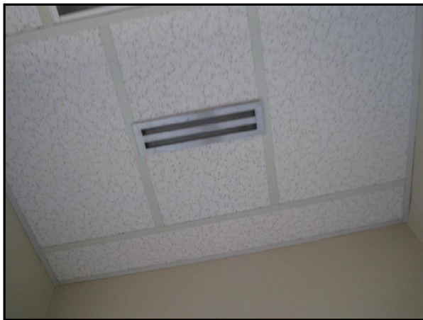
Distribution Systems - HVAC Ductwork Dirty
