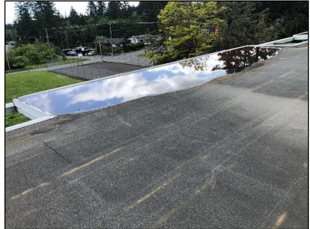
Photo 2 - Significant ponding
