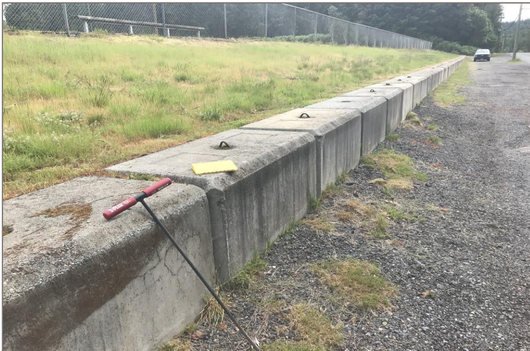
Photo 2: Lock Block Wall at Base of Site
