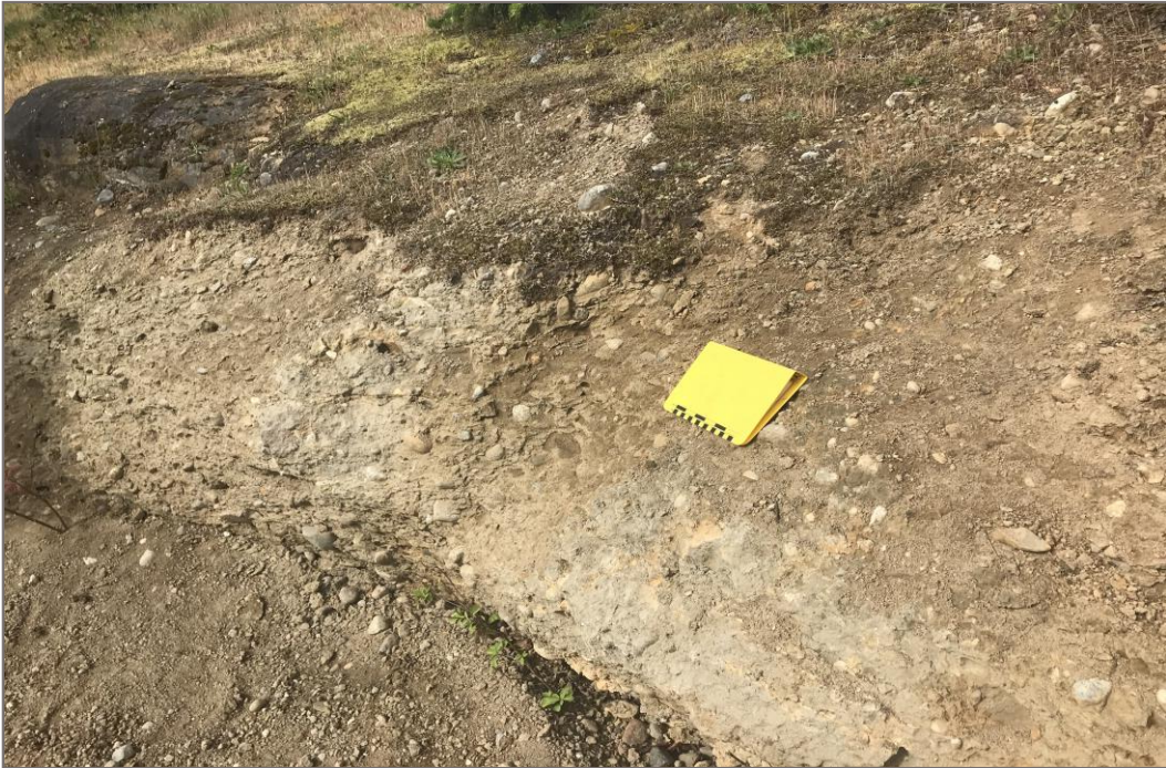
Photo 1: Soil Outcrop On Site Slope
