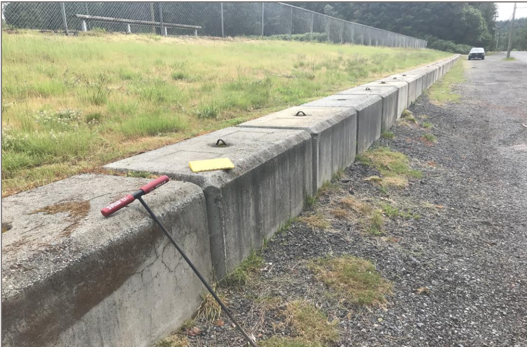
Photo 2: Lock Block Wall at Base of Site
