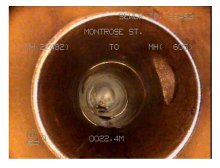
Figure 10. A sewer in almost perfect condition where infiltration is unlikely to occur
