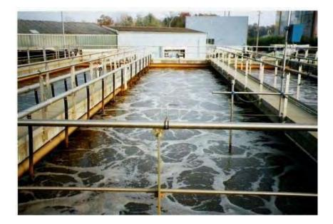
Figure 1 An Activated Sludge Aeration Tank
