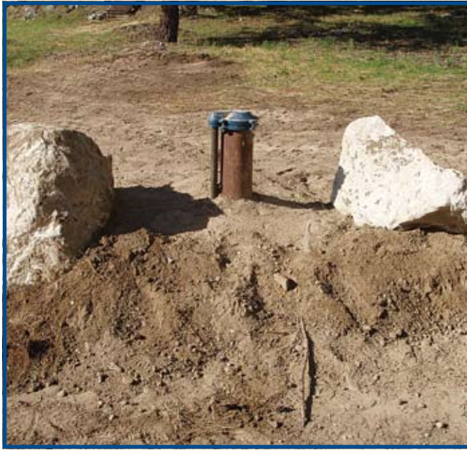
Figure 8. Grading around well head to protect well
