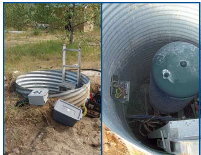
Figure 2. Well pit with metal cribbing
