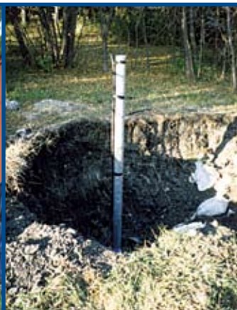
Figure 5. Well casing extended above ground level
