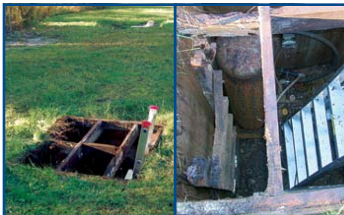
Figure 1. Well pit with wooden cribbing
