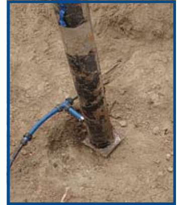
Figure 6. Pitless adapter installed below frost line
