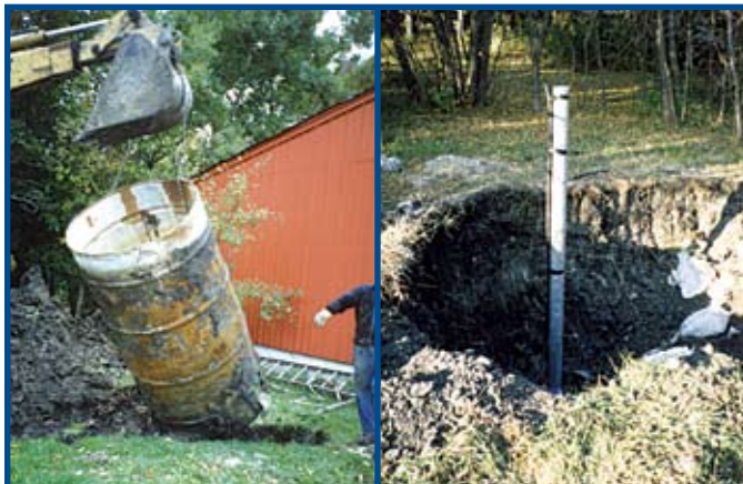
Figure 4. Well pit cribbing being removed by a backhoe
