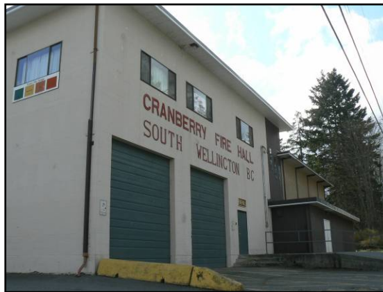
Cranberry Fire Hall – South Wellington
