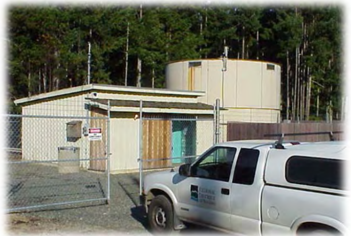
Melrose Pumphouse and Reservoir
