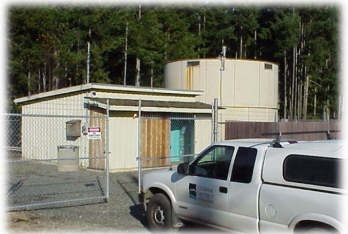
Melrose Pumphouse and Reservoir
