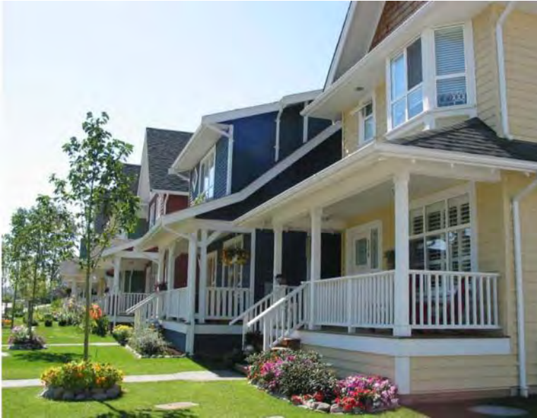
Alley loaded single family dwelling
