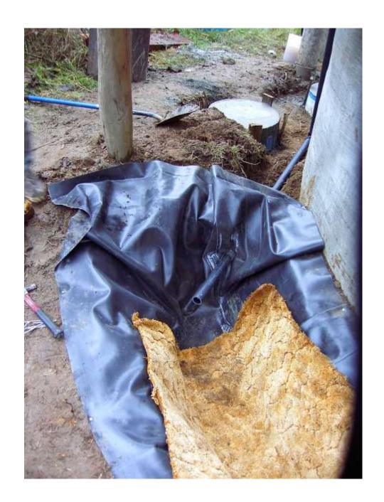
Drain port with overflow standpipe
