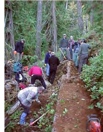
Volunteer maintenance crews at work (Photo: P. Rothermel).
