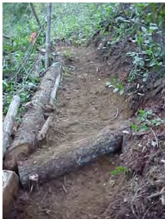
Completed erosion control measures (Photo: P. Rothermel).
