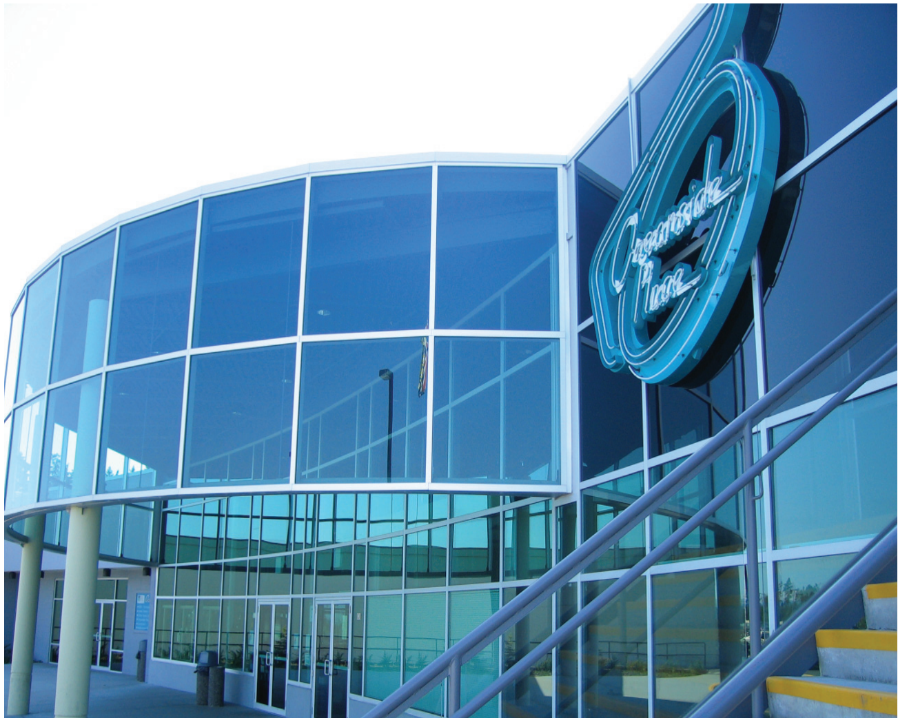
Oceanside Place is a two-sheet ice arena that was opened in October 2003 in the City of Parksville. Heat exchange on the ice plant should be explored in the immediate future
