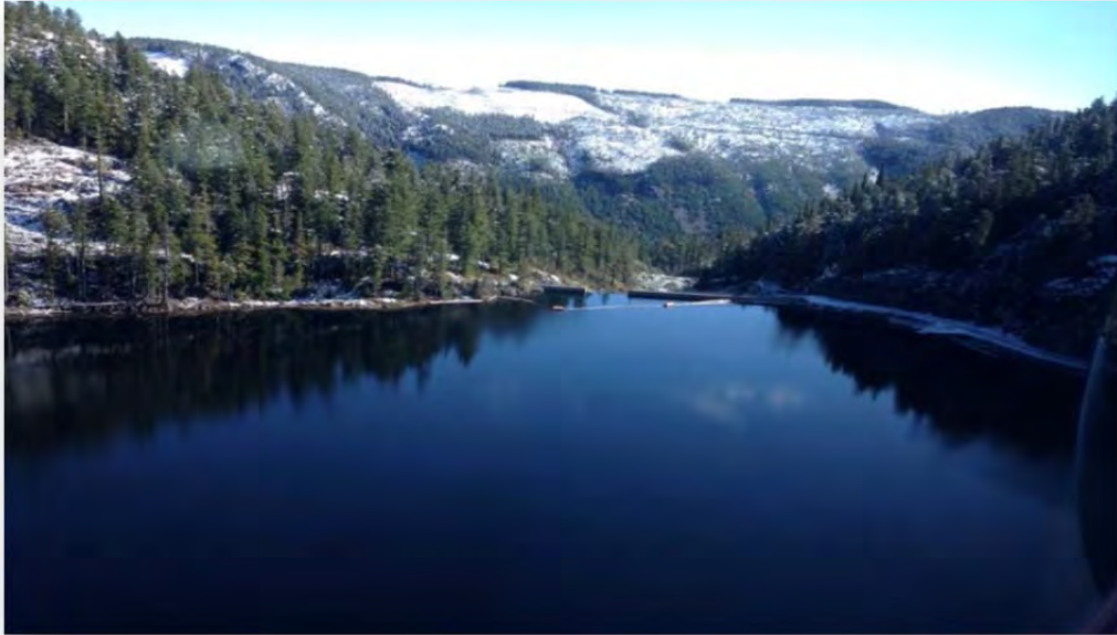
Arrowsmith Dam April 2014
