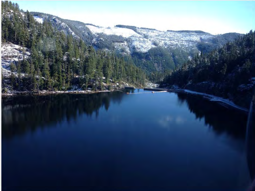
Arrowsmith Dam April 2014
