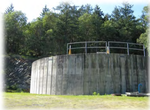
Photo of Fairwinds Reservoir No. 1
