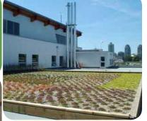
A green roof provides stormwater management and reduces heat island effect
