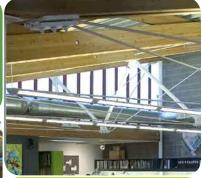
Coating added to clerestory windows filters the sunlight and reduces glare on computer monitors
