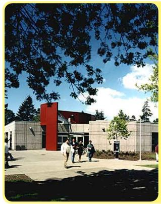
• This building has no mechanical cooling. Cooling is achieved with natural ventilation and strategies to reduce solar heat gain
