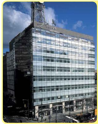
• This unique double skin feature helps to control the energy use within the building by contributing to natural ventilation and acting as a buffer for the very hot or cold exterior temperatures
