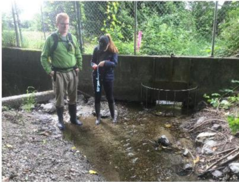
1.) Reach 3: Looking downstream at the diversion structure
