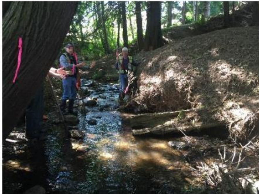
2.) R8 - Storm Water erodes historic stable banks
