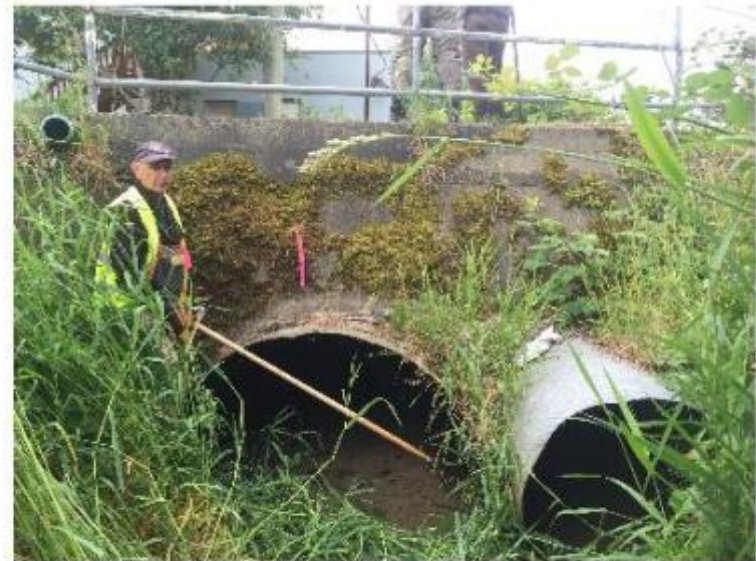
4.) Bay St twin culverts are smaller but passable..
