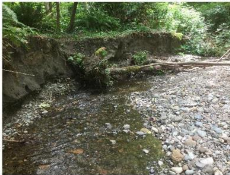
2.) Reach 4: Bank Erosion site at riffle 6
