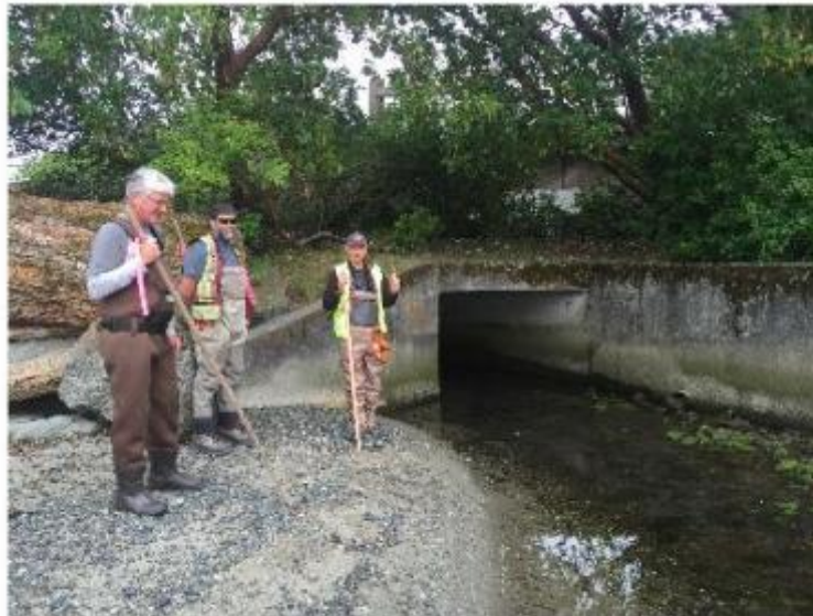
2.) Departure Road culvert is fish friendly
