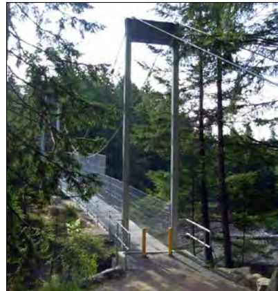
Example of completed Suspension Bridge (photo: Harold Engineering)
