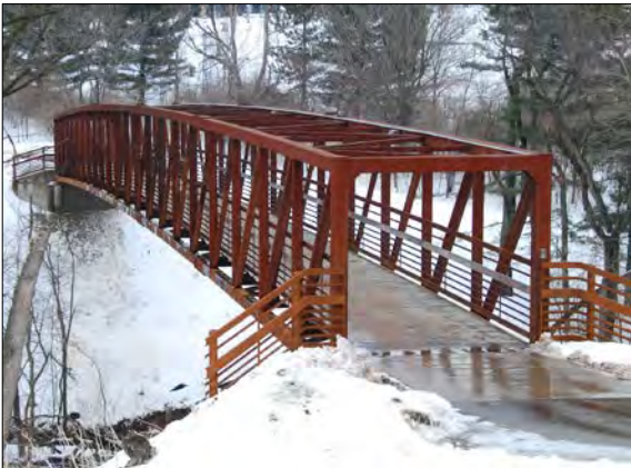
Example of completed Steel Truss Bridge (photo: Harold Engineering)
