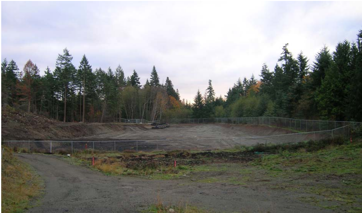
Figure 3. East view of GNPCC site cleared for proposed secondary treatment plant construction
