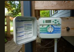
Typical Residential Irrigation Controller
