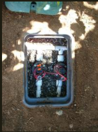
RCVs in Valve Box
