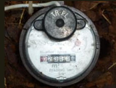
Water Meter Reading
