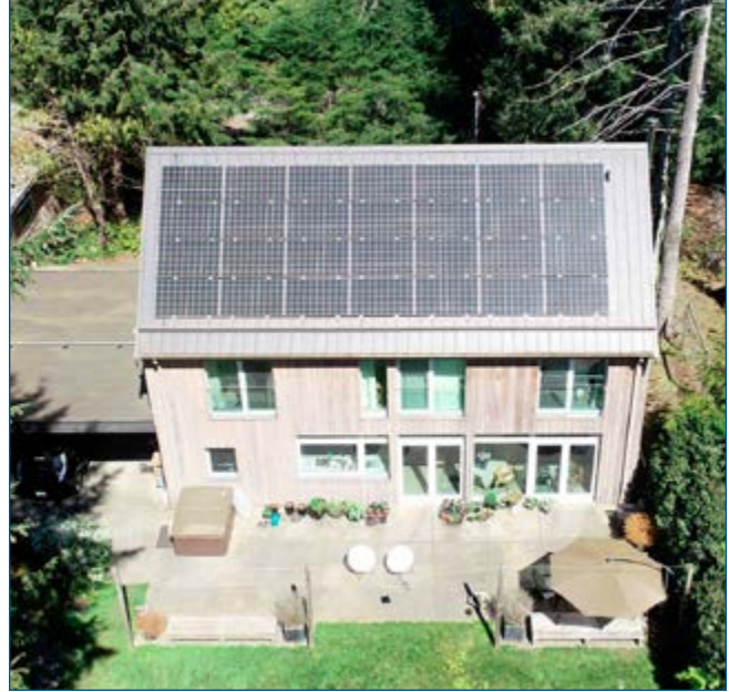
Home in Black Creek, BC sited for maximum solar gain. Overhangs can be added to reduce solar gain in summer.
