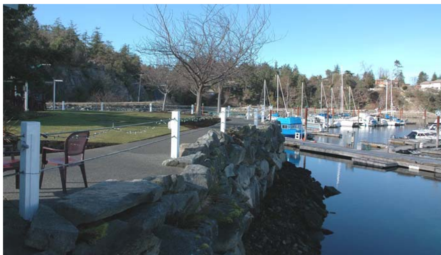
Figure 5: Grassy picnic area (Segment 2) showing vertical block wall and riprap fill.
