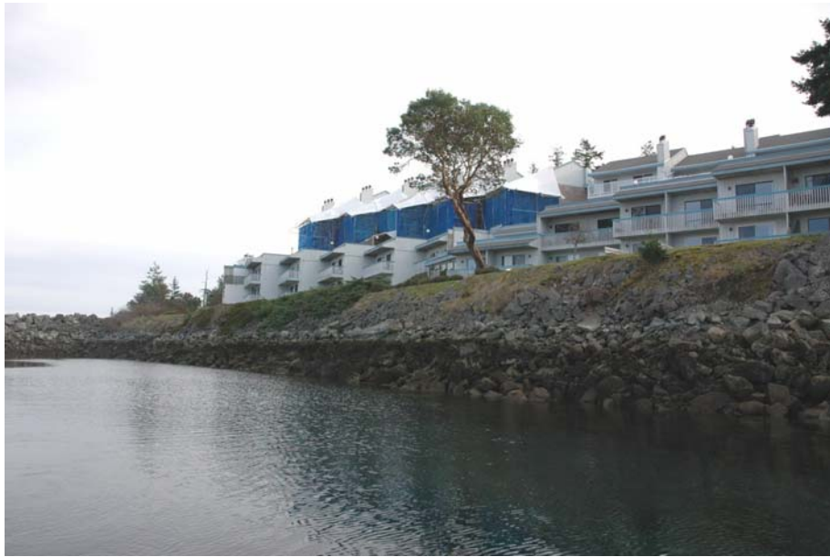
Figure 11: View of steep bedrock and fill shoreline in Schooner House segment.
