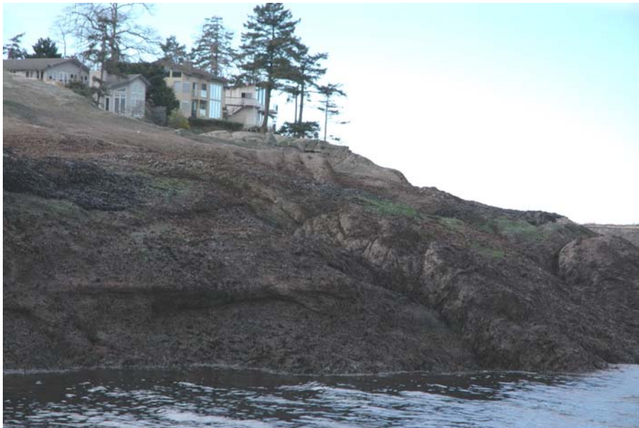
Figure 26: Bedrock ramp at north entrance to Schooner Cove. This section of the segment would be classified as semi-exposed wave energy.
