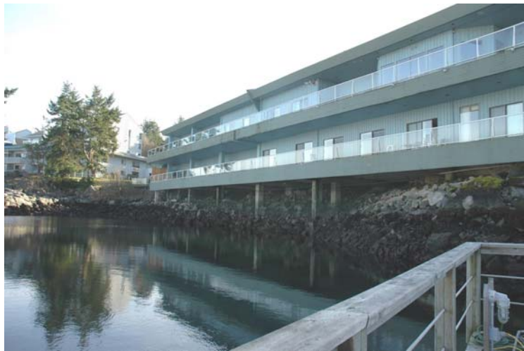
Figure 7: View of hotel building, showing pilings over the intertidal zone.
