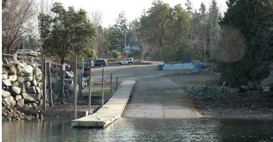
Figure 3: View of beach, boat ramp and marine ways in Segment 1, showing paved concrete ramp, floating dock, metal piles of the marine ways. Transect T1 was surveyed across the beach area at the right of this photo.
