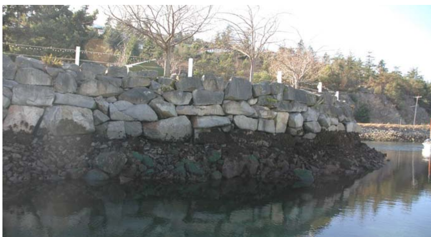
Figure 6: Shore Segment 2, with rockweed and green algae along the lower wall and riprap fill.
