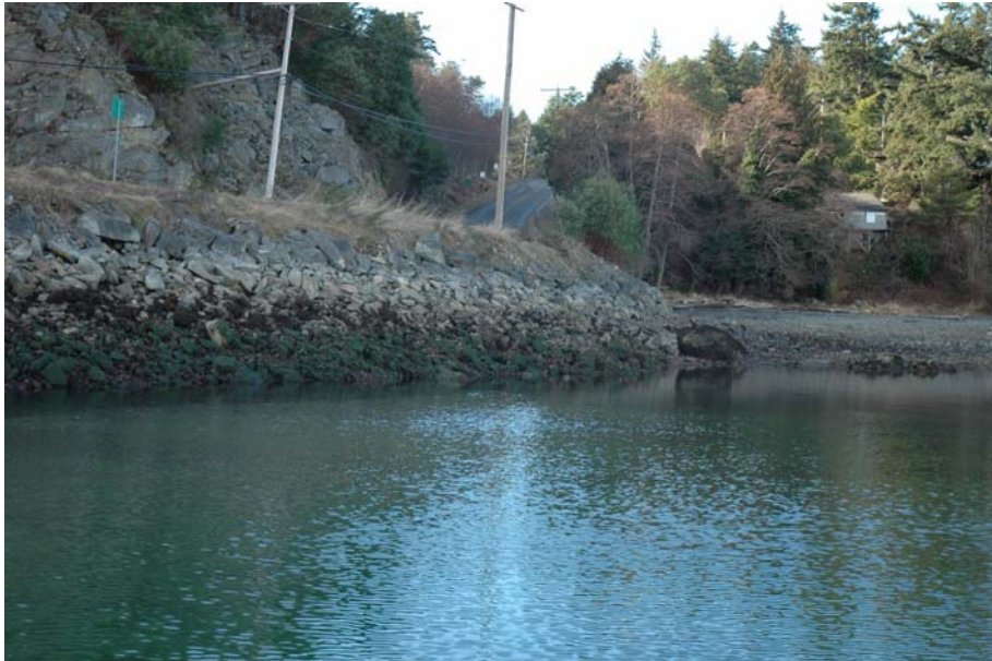
Figure 27: Steep riprap road bank at the west end of Schooner Cove in Segment 9.
