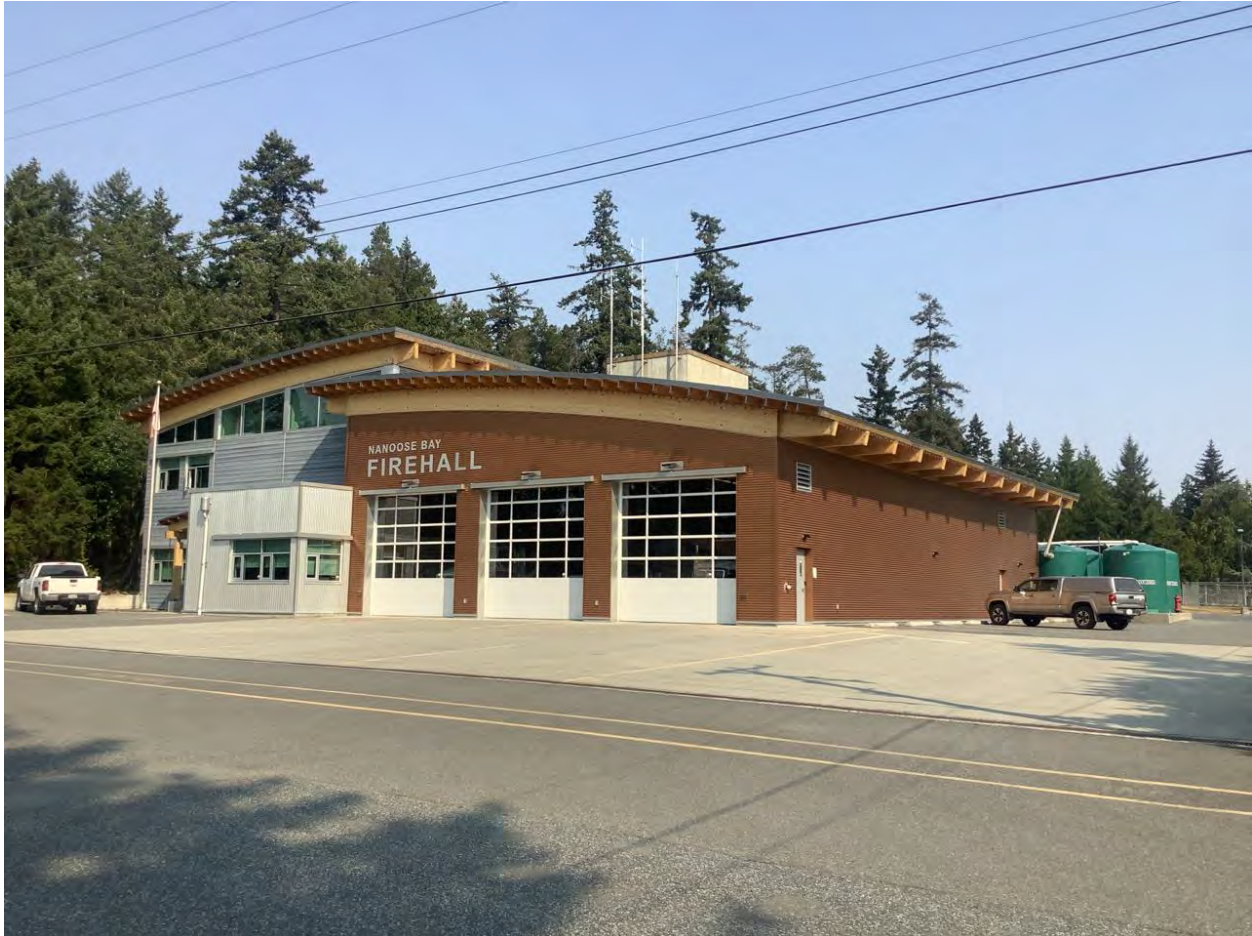
Photo 7. Nanoose Bay Fire Hall is an example of FireSmart construction that incorporates wood elements.
